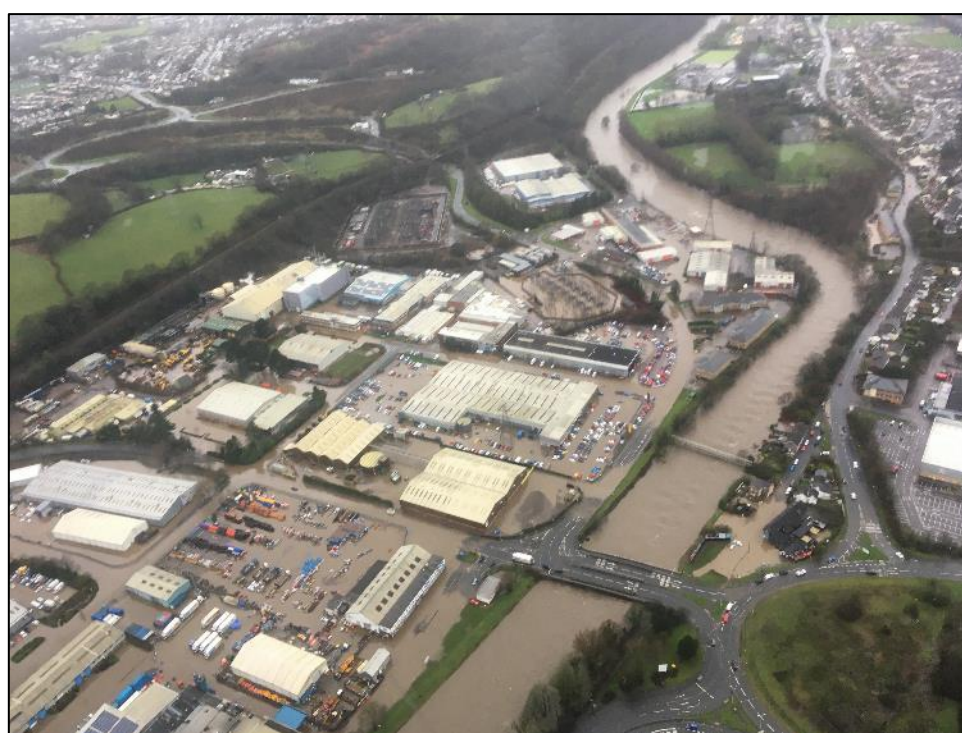
Figure 3: Aerial view of Treforest Industrial Estate and Upper Boat following Storm Dennis (Image: National Police Air Service)
